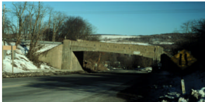
The reinforced concrete grade separation structure illustrated was built in 1938 to carry a local street over the Lincoln Highway's Stoystown Bypass in Pennsylvania. It was designed with access ramps, and stands as a rare example of a pre-World War II interchange.
