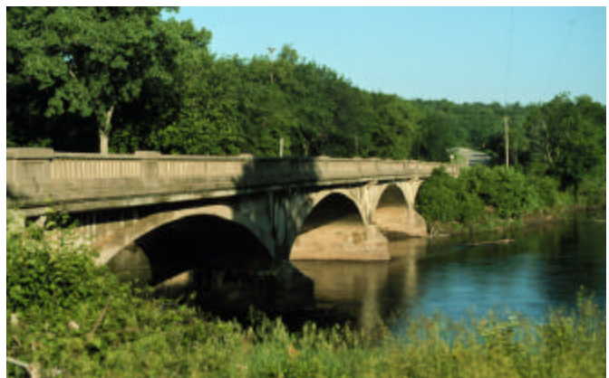
The 1913 Eureka Bridge is a multiple span, closed spandrel reinforced concrete arch bridge over the North Raccoon River west of Jefferson, Iowa.
