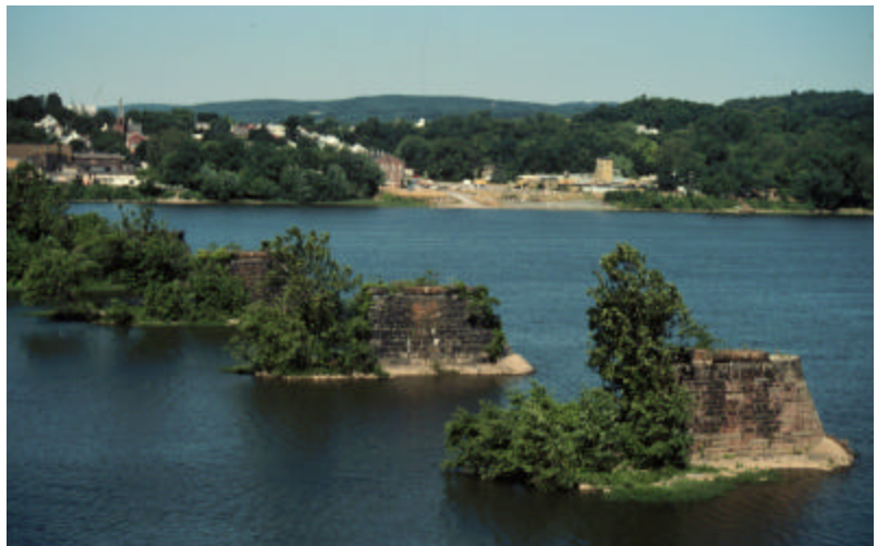
Bridge piers and abutments to now gone spans can also be important resources to the interpretation of the historic Lincoln Highway. These stone piers in the Susquehanna River supported the combination Pennsylvania Railroad and Lincoln Highway bridge before the opening of the Intercounty Bridge.
