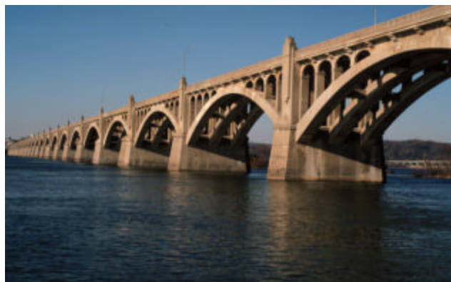
The 1930 Lancaster-York Intercounty Bridge over the Susquehanna River is one of the few remaining large span Lincoln Highway bridges from the period of significance.
