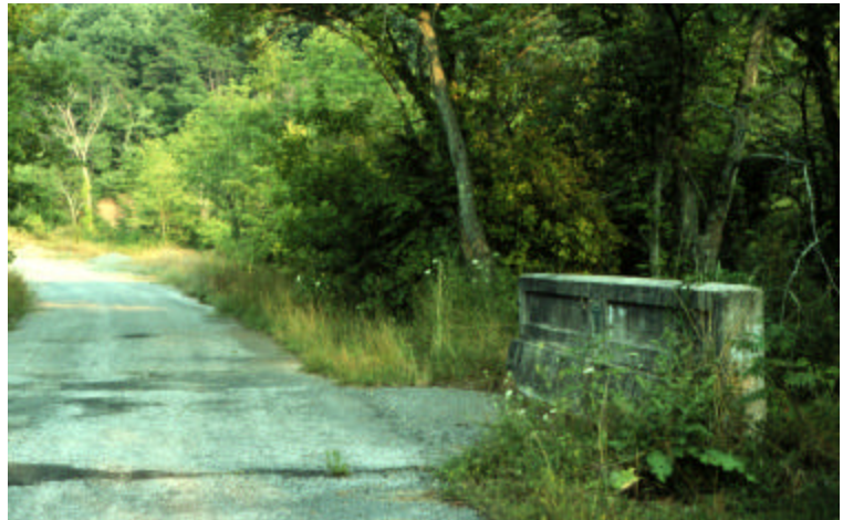
This Lincoln Highway remnant east of Schellsburg, Pennsylvania, retains its early concrete pavement, width, and culvert with a 1917 date plate.
